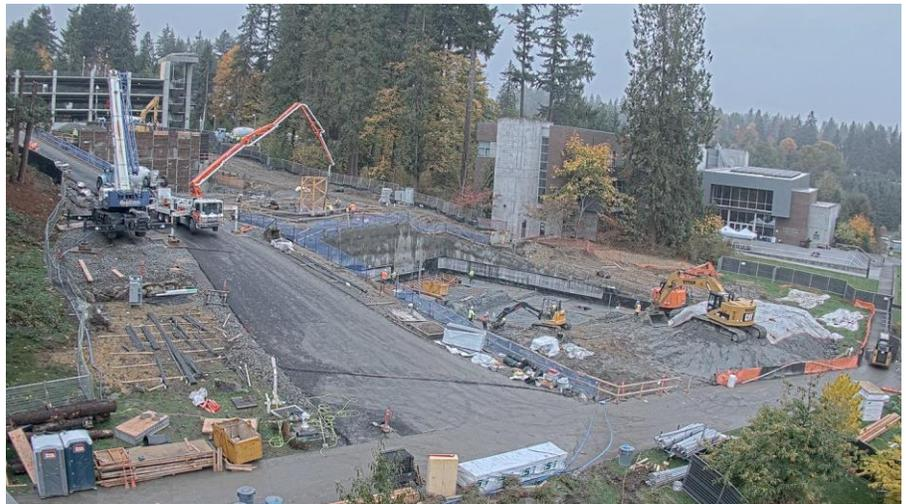
Foundation work has begun with placement of the Tower Crane Footing (shown in photo above). Foundation work including waterproofing, rebar, and concrete will continue at Level 0 with the perimeter footing giving shape to the footprint of the buildings lowest level that will exit out onto the Crescent Path. Foundation work will then elevate to the next step, creating Level 1’s footprint.
